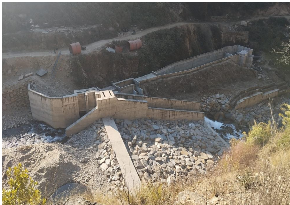
Figure 6-1: Figure 6 1: Head Works Structure
