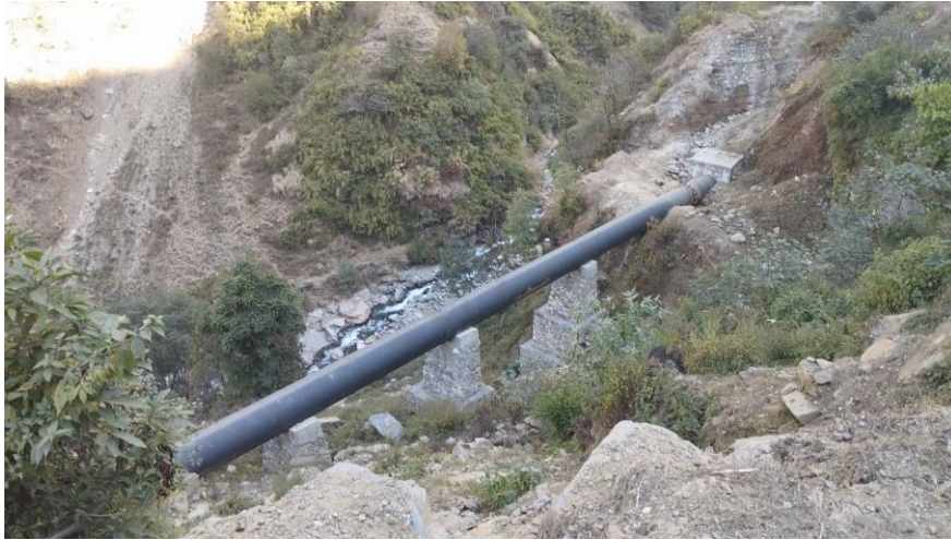
Figure 7-3: Stone Masonry Saddle Support.
