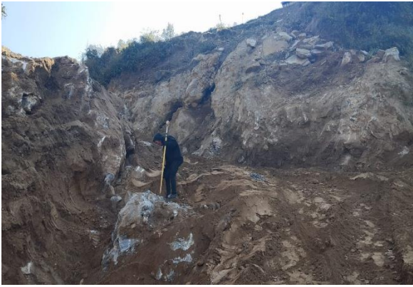
Figure 8-3: Surge Shaft Ongoing works
