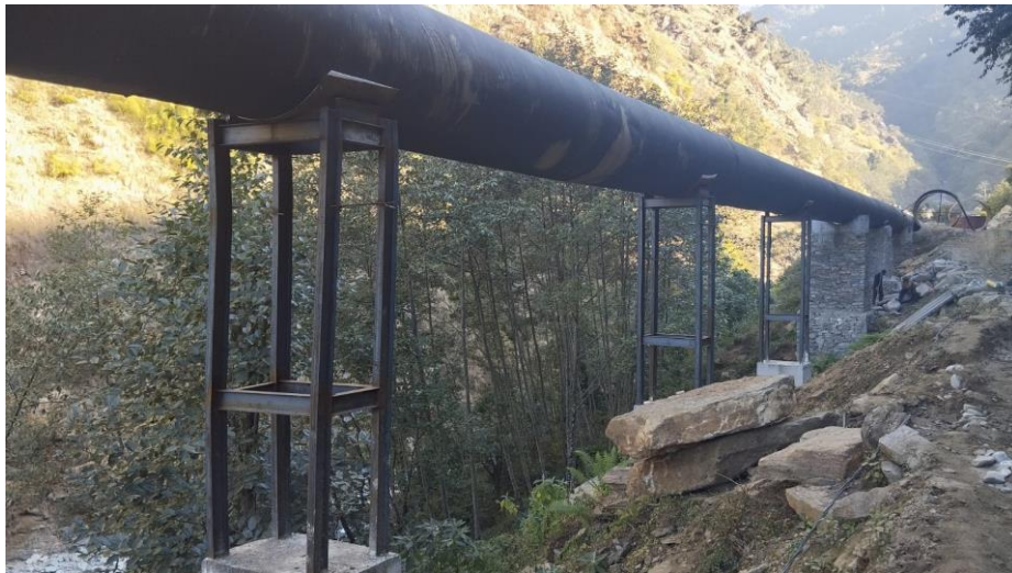
Figure 7-2: Steel I-Section Saddle Support.
