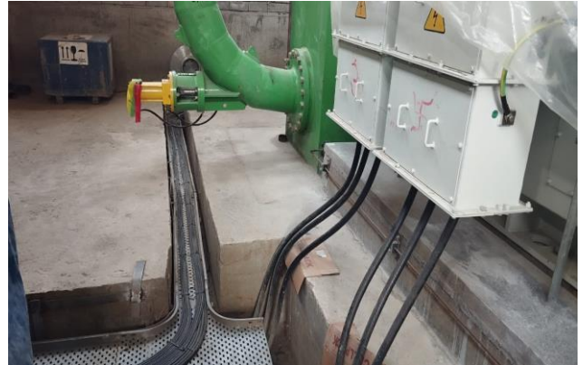
Figure 9-3: Powerhouse Machine Foundation
