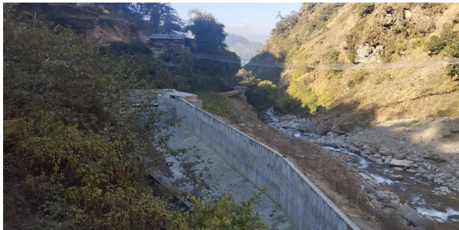
Figure 6-3 : Settling Basin.
