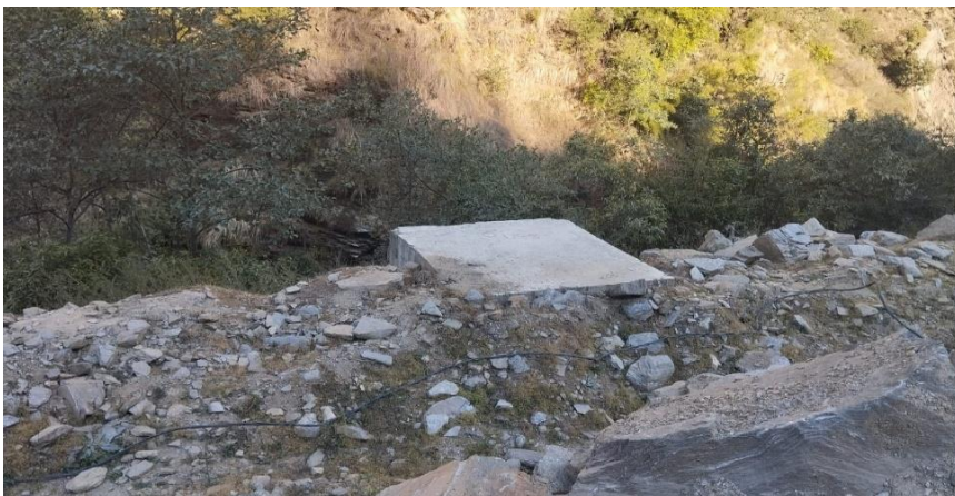
Figure 7-5: Anchor Block.
