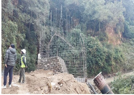
Figure 8-4: Anchor Block (AB=31A)
