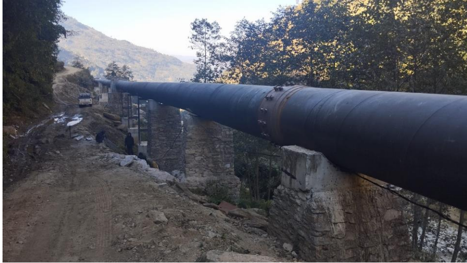
Figure 7-1: Head Race Pipe Erection.
