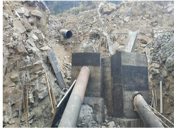
Figure 8-3: Bifurcation branch pipe
