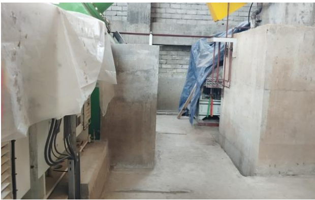
Figure 9-2: Powerhouse Machine Installation
