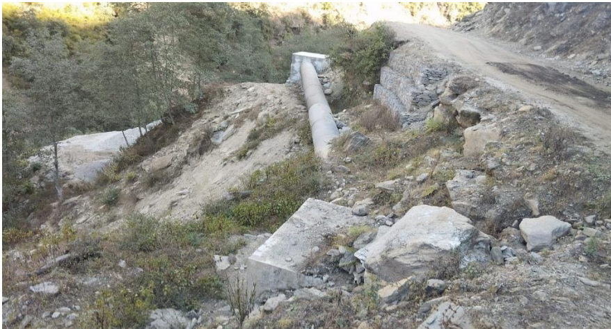
Figure 7-4: Head Race Pipe.
