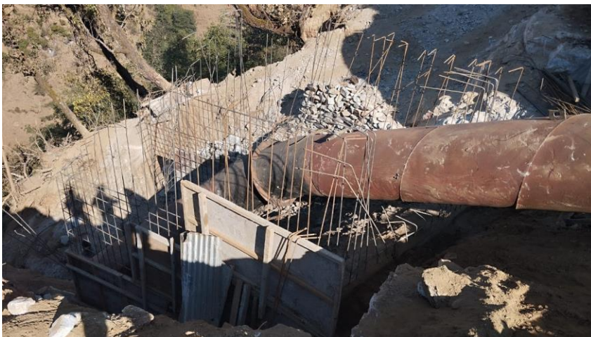
Figure 8-2: Anchor Block (AB-31).
